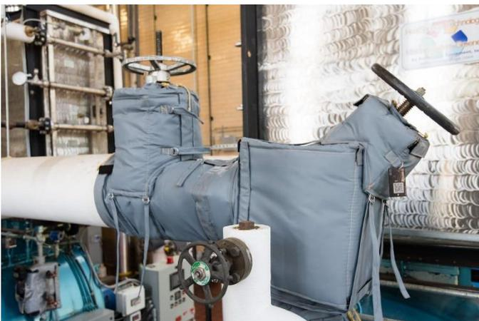
Figure 9-2 Insulation jacket over valves, Source: [www.thermaxxjackets.com](http://www.thermaxxjackets.com)
