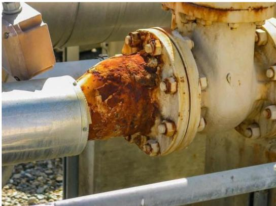
Figure 8-7 Result of the steam leak, Source: David Seibold on flickr.com, CC-BY-NC 2.0
